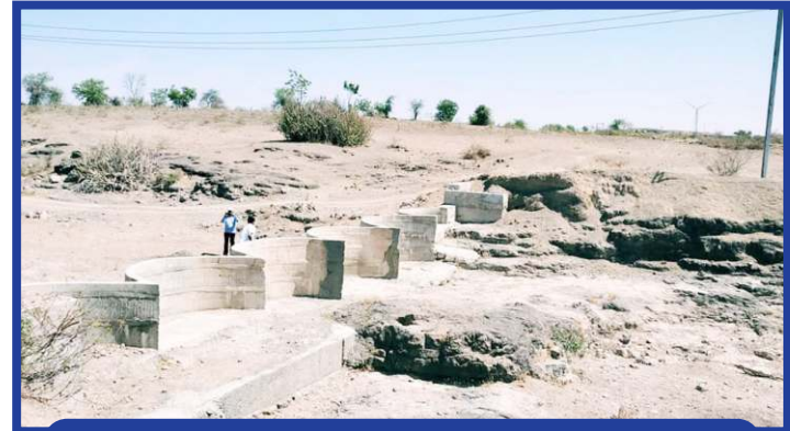
Ferrocement Dam prepared by Reliance Foundation
